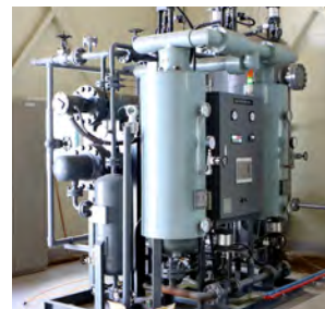
Dryer for High pressure air
