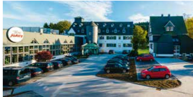
Headquarters of Jokey Plastik Wipperfürth GmbH Germany
